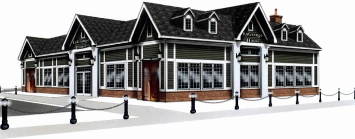
Restaurant – rear and parking lot view
