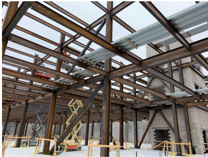
Active Construction at Incyte
