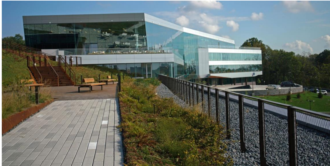
Green roof at Incyte
