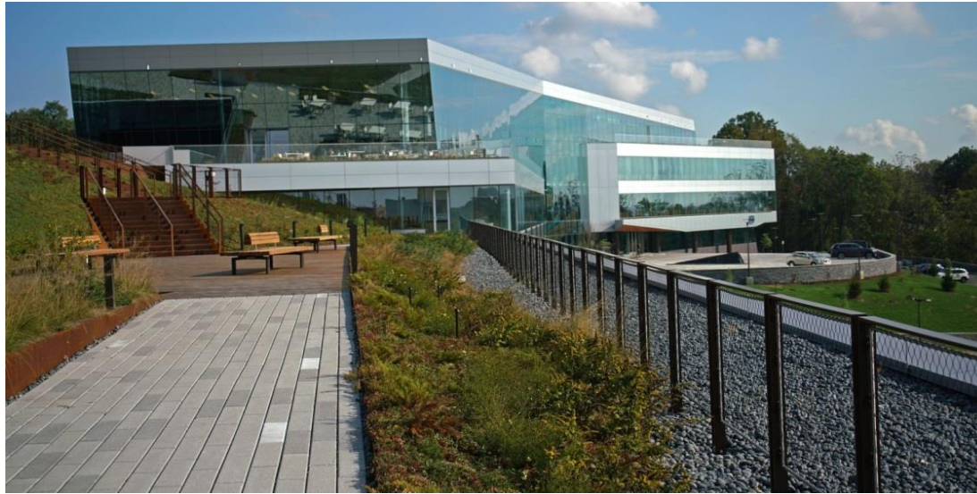
Green Roof at Incyte
