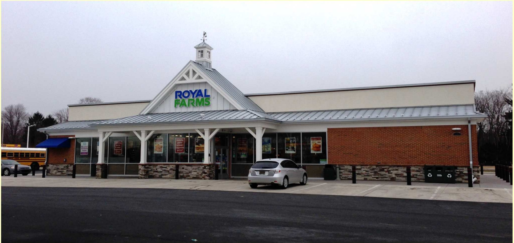
5100 SF Convenience Store with Gas Pumps for Royal Farms in Wellington Commons
