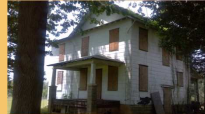
2493 Sunset Lake Road, Glasgow Park Demo Application Underway
