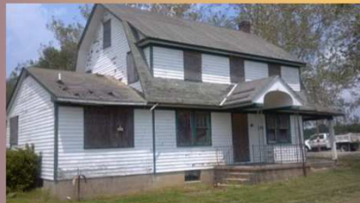
2493 Sunset Lake Road, Glasgow Park Demo Application Underway
