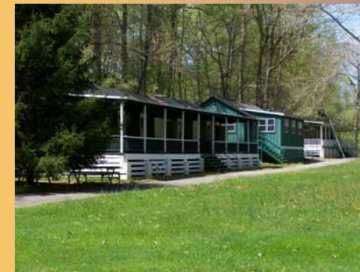
3850 Mill Creek Road Camp Wright Demo Application Underway
