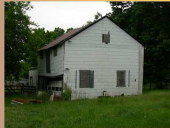
Jester Property OutBuilding 2818 Grubb Rd
